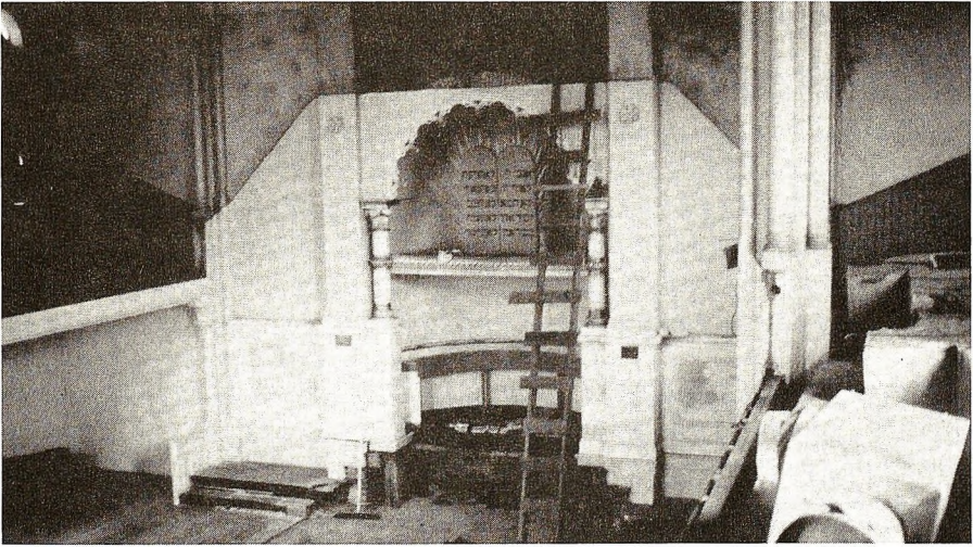
Interior after restoration begun and false ceiling removed
