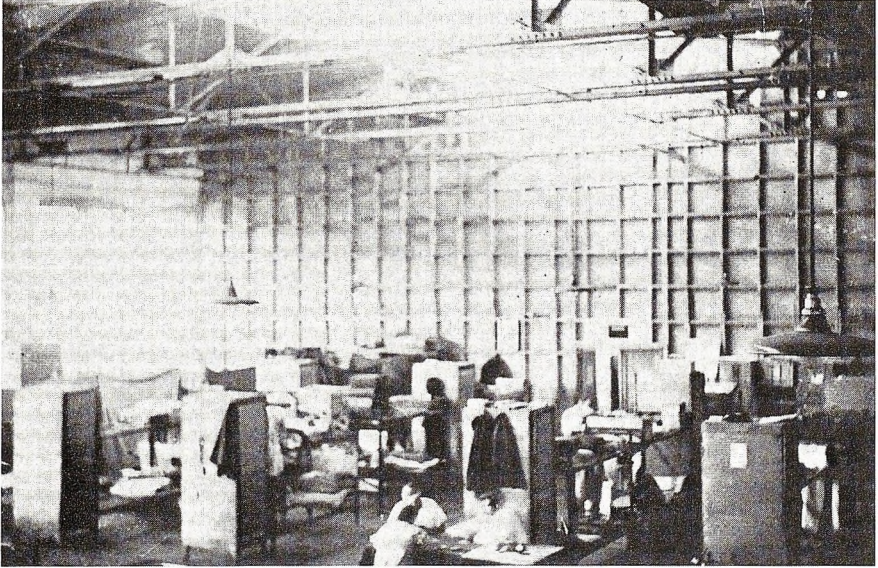
Figure 3: Camp "N" - Interior view (Courtesy of Public Archives of Canada)
